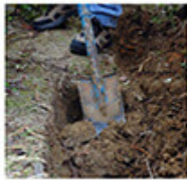
LAY OUT SYSTEM, DIG TRENCHES AND HOLES
