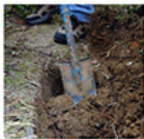
LAY OUT SYSTEM, DIG TRENCHES AND HOLES
