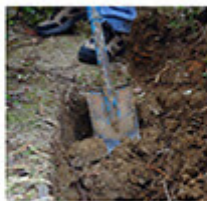
LAY OUT SYSTEM, DIG TRENCHES AND HOLES
